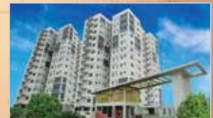
The Arena Haldia International Sports City, Haldia
